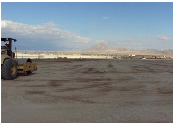
CAMU: Phase II and Phase I grading for liner subgrade.
