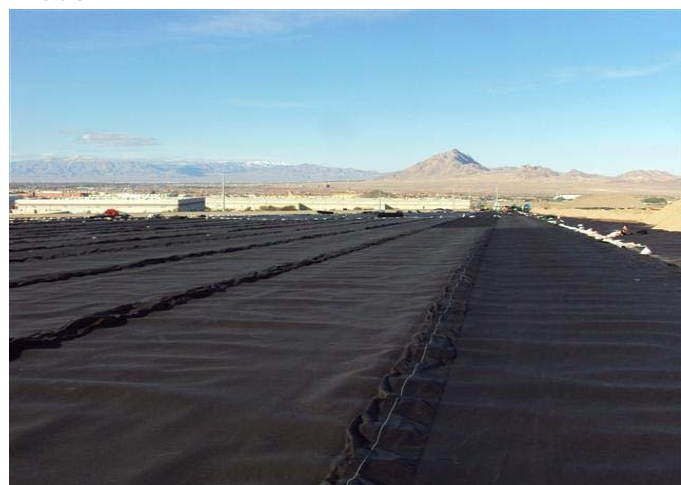
CAMU: Phase I and Phase II, geocomposite.
