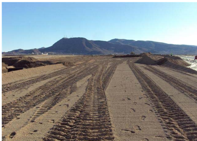
CAMU: Phase I and Phase II, final cover soils.
