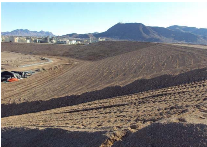
CAMU: Eastslope, Phase I and Phase II. Final cover soils.
