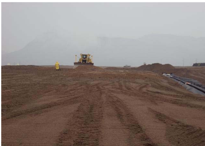
CAMU: Phase I, Phase II and Phase IIIB. Placing final cover soils.
