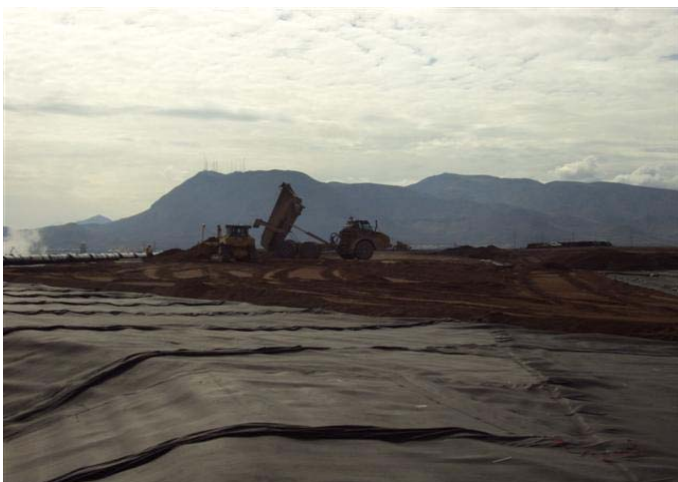
CAMU: Phase I, Phase II, and Phase IIIB, final cover.
