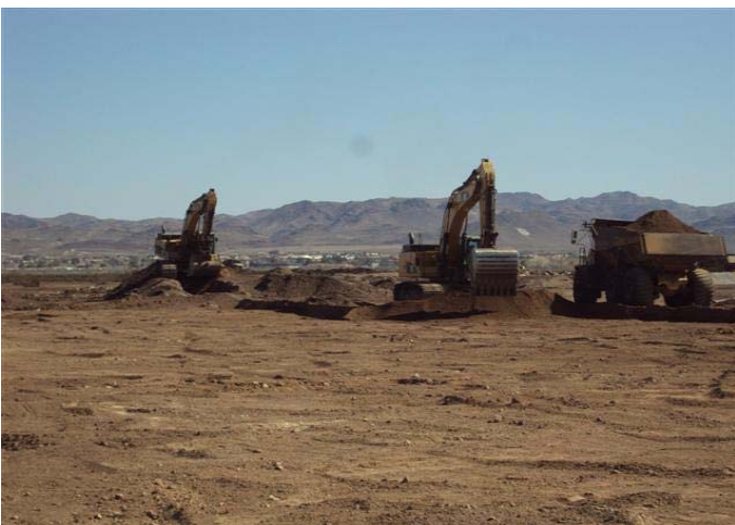
Eastside: Haul road and laydown area scrape.
