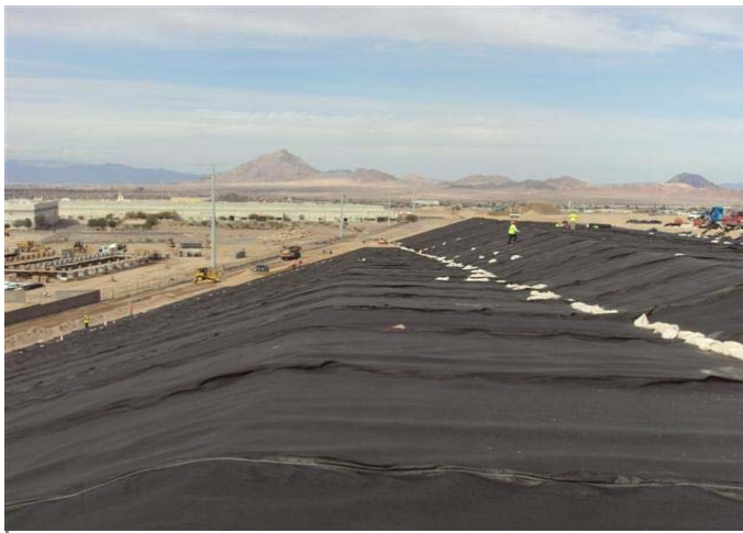
CAMU: West slope. Geocomposite.
