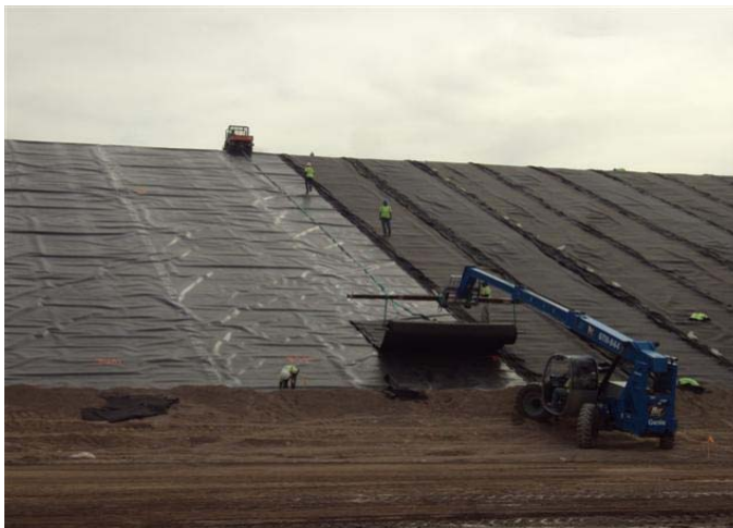
CAMU: Phase IV, north slope, geocomposite.
