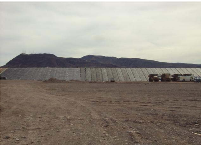
CAMU: Phase IV, north slope, geocomposite.
