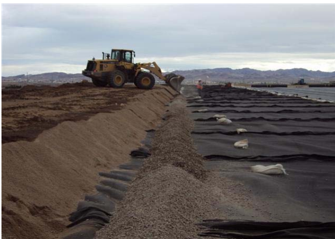
CAMU: Phase IV, top, CPE drainage rock.
