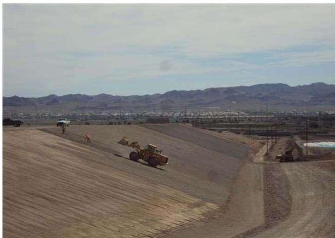
CAMU: Phase IV, south slope, installing gravel mulch.
