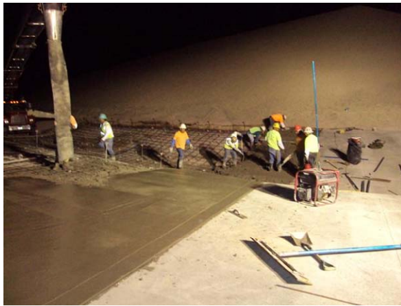
CAMU: South west channel, concrete finishing.
