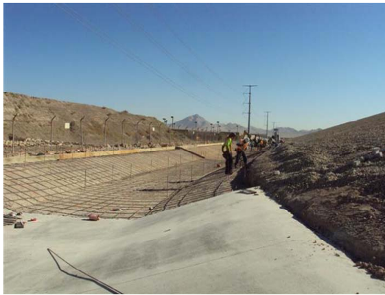
CAMU: West channel, concrete preparation.
