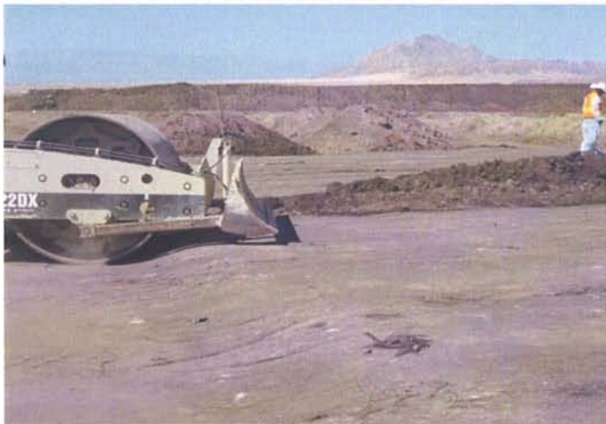
Eastside: Roller used to provide compaction.
