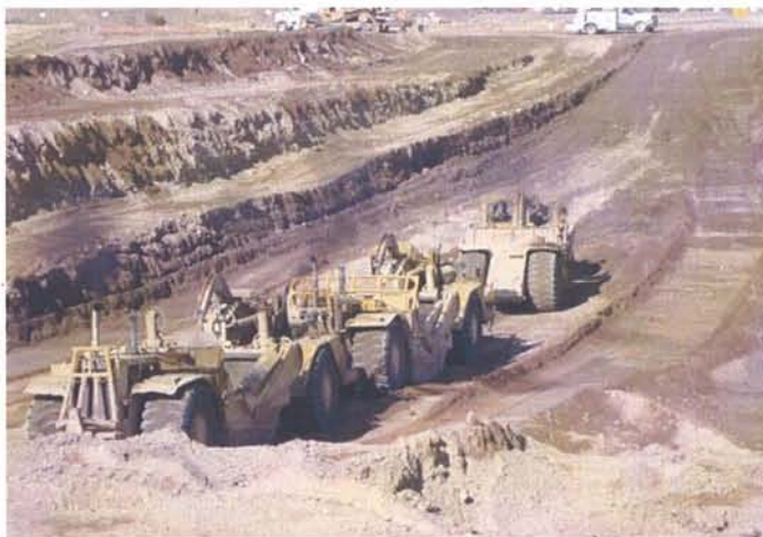
CAMU: Phase 1 clean soils north of western ditch being removed by Scrapers..
