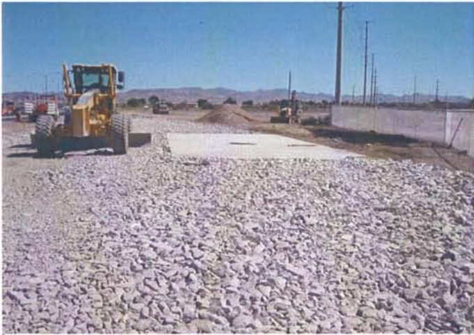
Westside: Decon trackout rock placed.
