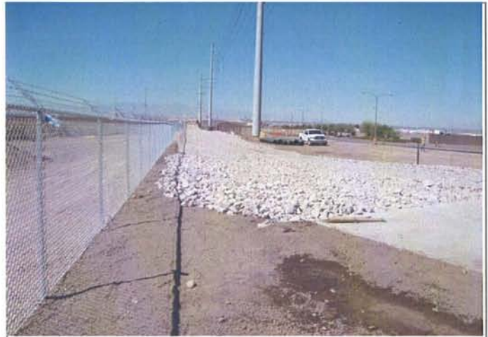
Westside: Trackout rock placed
