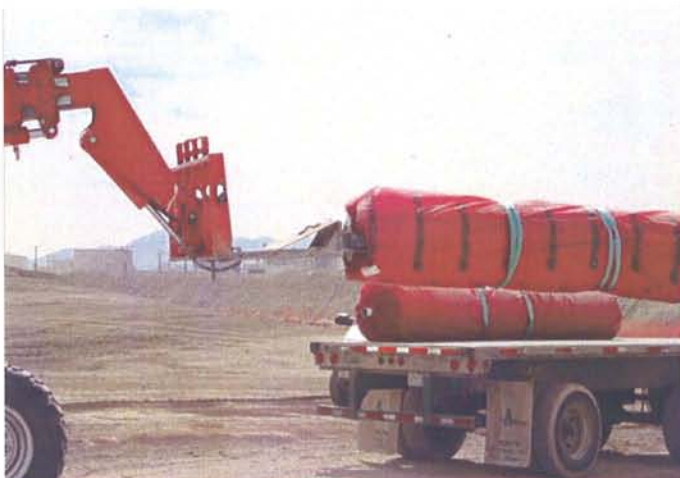
CAMU: GCL liner being offloaded with a stinger pole.
