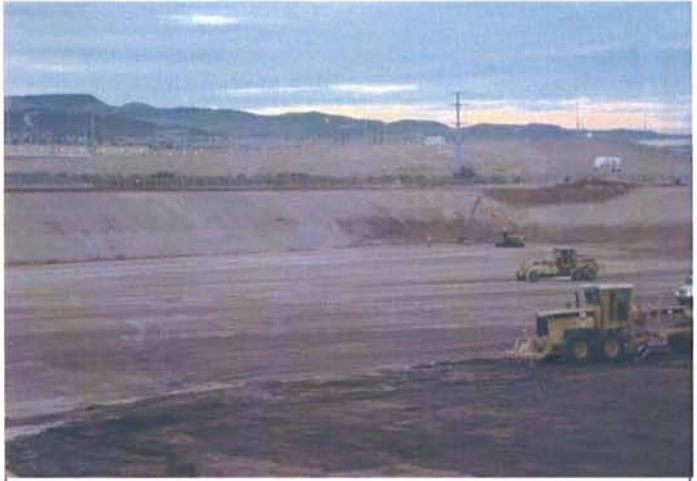
CAMU: Phase II southeast corner beginning rolling the slopes at dawn.
