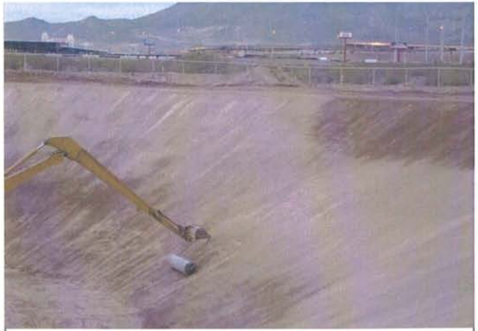
CAMU: Phase II subgrade on slopes being rolled.
