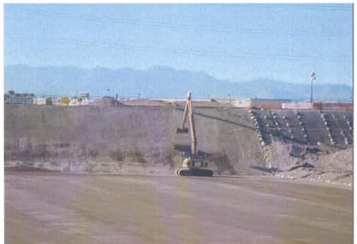
CAMU: Phase II, western ditch west slope being rolled.
