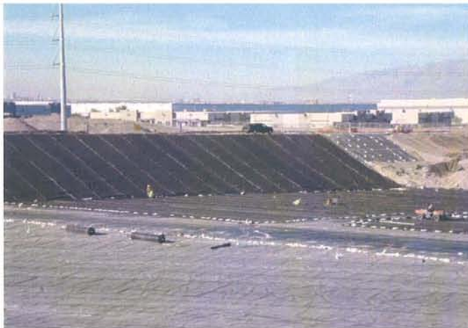
CAMU: Geocomposite installation of west slope at Phase I tie-in. Proceeding south in Phase II.
