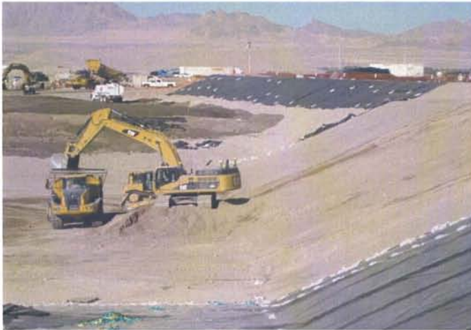
CAMU: Western ditch, east slope shaping and ramp removal.
