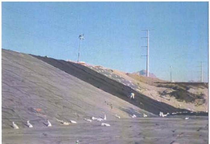
CAMU: Geocomposite installation west slope beginning Phase II.
