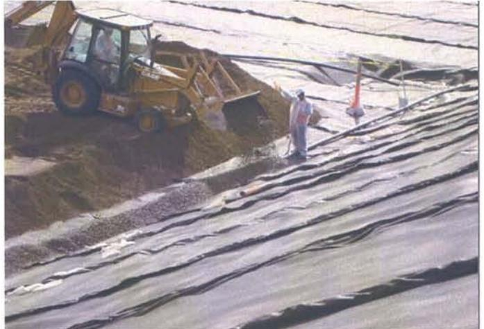
CAMU: Phase II, LCRS pipe, toe drain rock installation.
