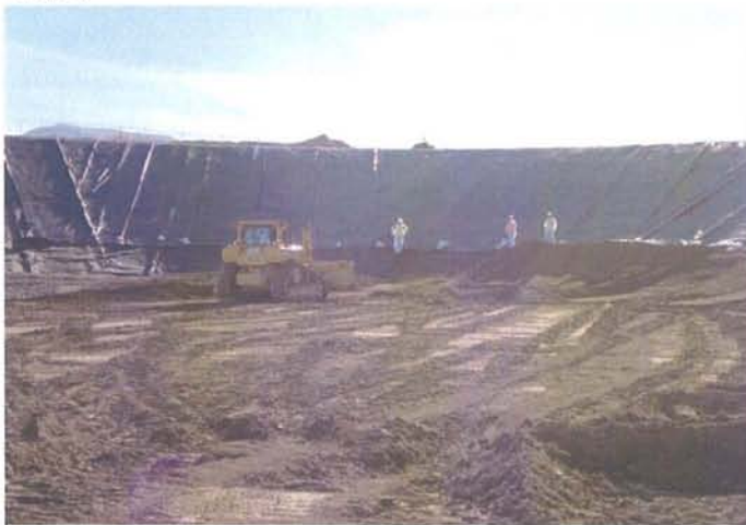
CAMU: Phase II Southwest corner placing operations layer on slope.
