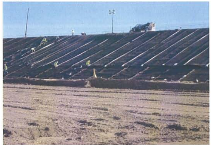
CAMU: Phase II South slope installing woven geotextile.
