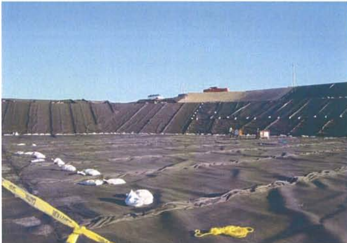
CAMU: Phase II, Geocomposite installed looking Southeast at Phase IIIA bench.
