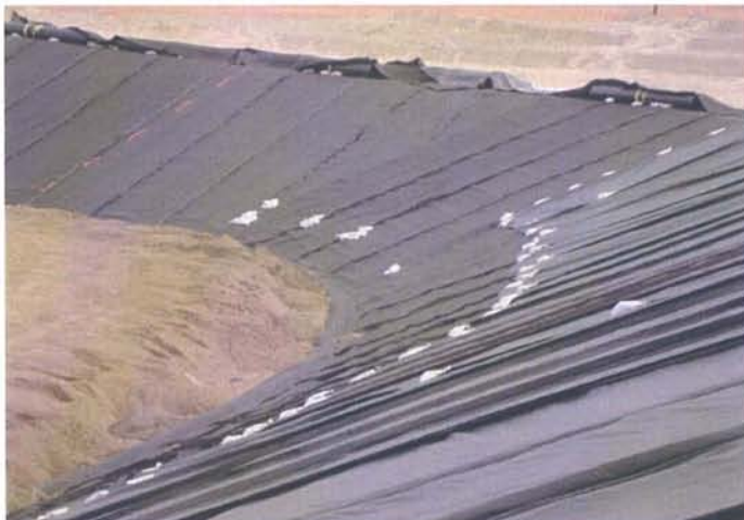
CAMU: Phase II Southeast corner toe drain installation.
