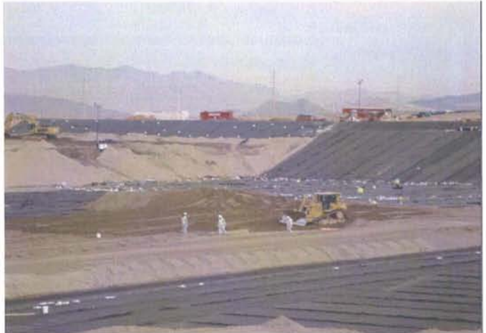
CAMU: Phase II, placing operations layer.
