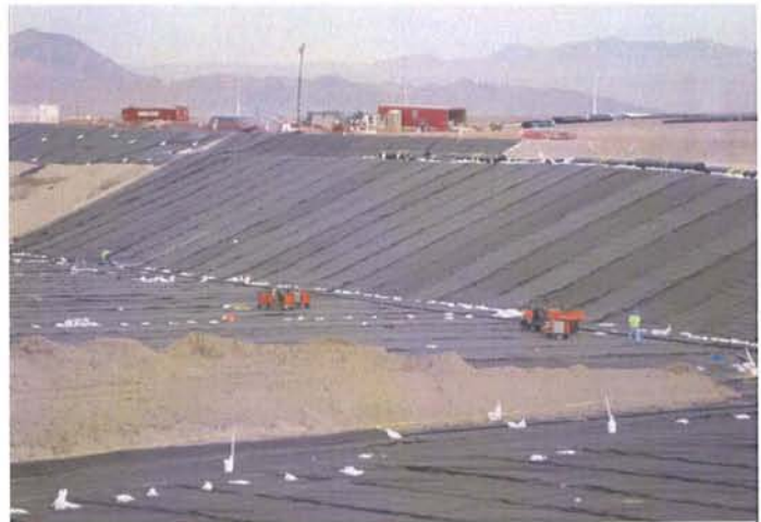
CAMU: Phase II, East slope and floor, geocomposite installed.
