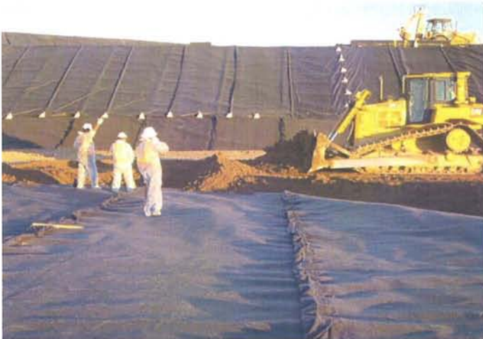
CAMU: Phase II, operations layer placement being monitored by Entact, Geosyntec, Weston.
