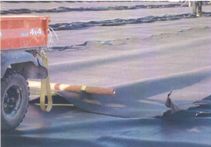
CAMU: BMI North Landfill deploying Geocomposite liner.
