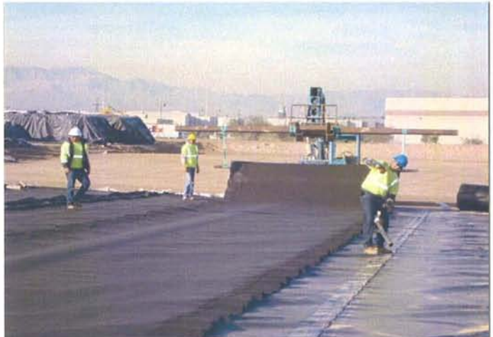
CAMU: BMI North Landfill, deploying Geocomposite liner.
