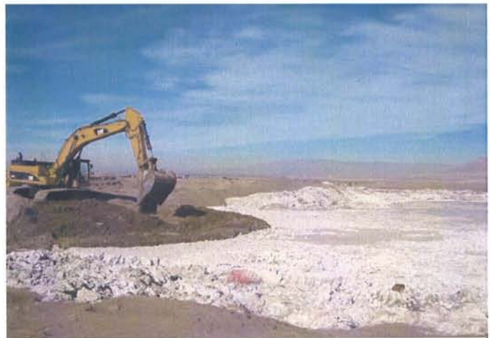
Eastside: SW-2, mixing dry soils with wet material.
