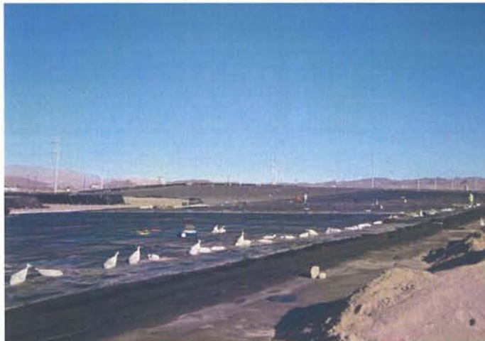
CAMU: North BMI Landfill liner installation.
