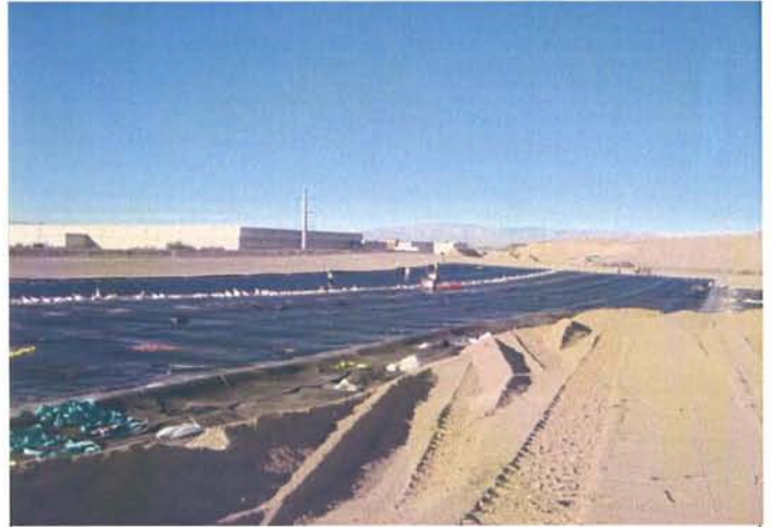
CAMU: North BMI Landfill liner installation.
