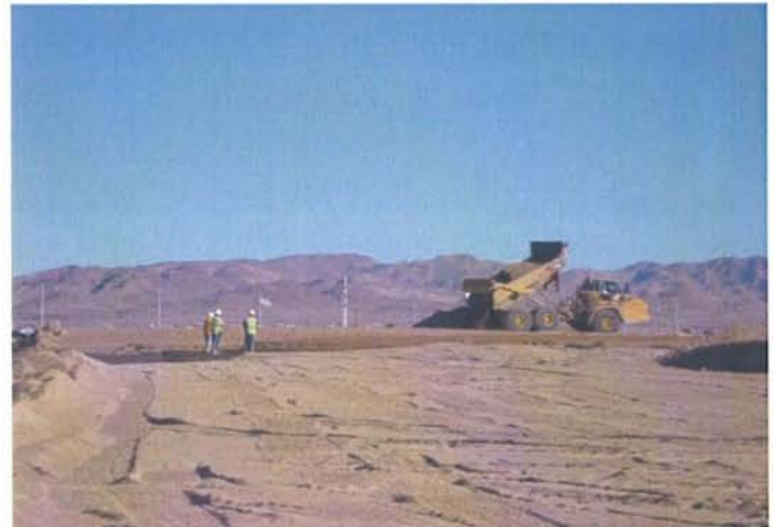
CAMU: North BMI Landfill, Entact, Geosyntec, and Weston monitoring the placement of 1" minus 12" layer on liner.
