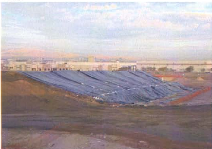
CAMU: Phase I, Visqueen placement North slope.
