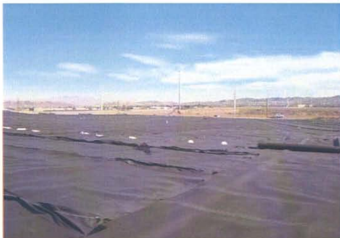
CAMU: North BMI Landfill, geocomposite liner installation, looking east.
