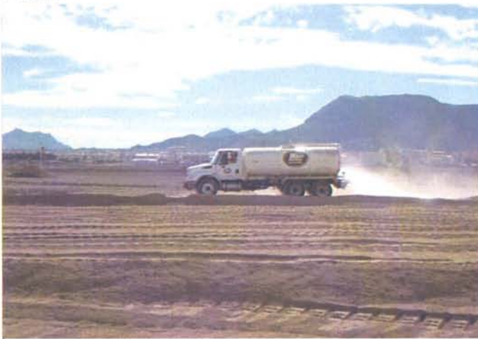
CAMU: North BMI Landfill, dust control on cover soils.
