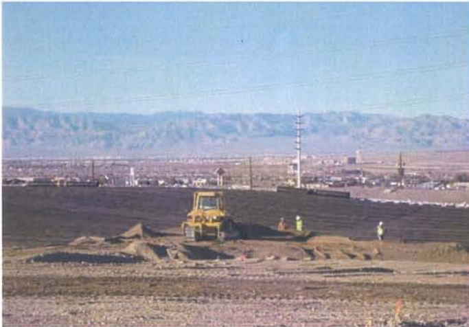
CAMU: North BMI Landfill, placing 1" soils.
