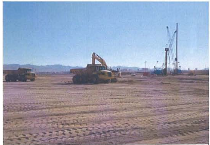
.CAMU: Slit trench excavation and sheet pile driving operation.
