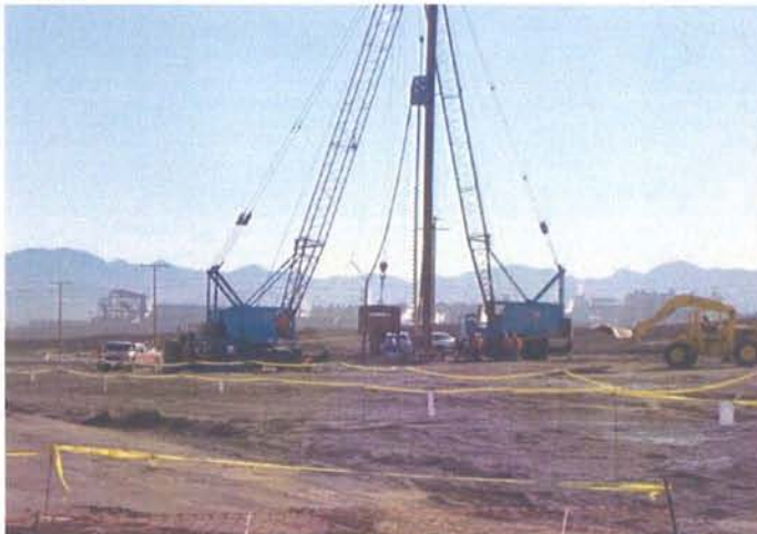
CAMU: Sheet pile driving operation.
