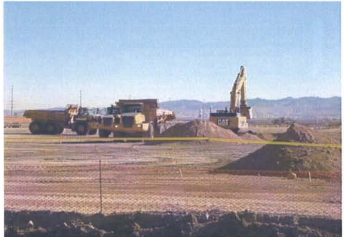
CAMU: Slit trench SLT4W, excavation.
