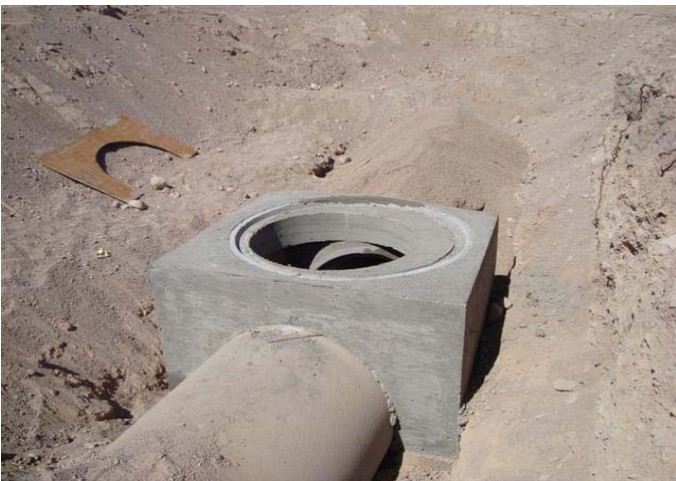
CAMU: Manhole # 4, Storm drainage system.
