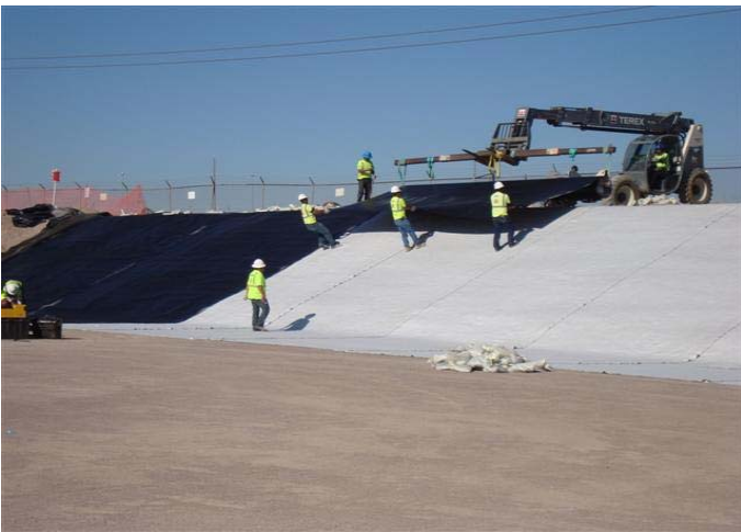
CAMU: Phase IIIB, Liner installation.
