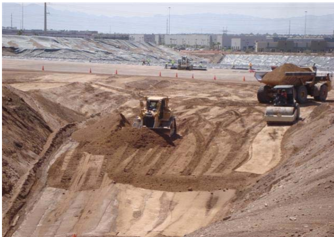
CAMU: NW-1, Slit trench. Backfilling.
