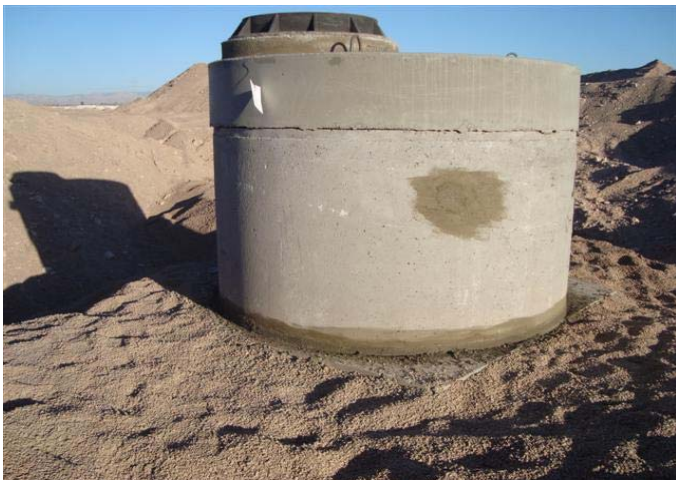
CAMU: Storm drain manhole.
