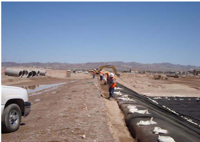
CAMU: Phase IIIB, anchor trench.
