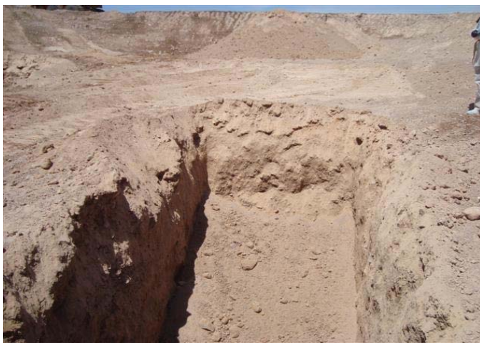
CAMU Inspection of trench NE-1, pothole is to design elevation.
