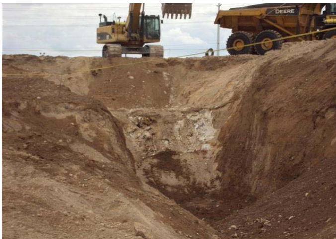
CAMU: NE-2, Slit trench. Waste beyond design limits. East.
