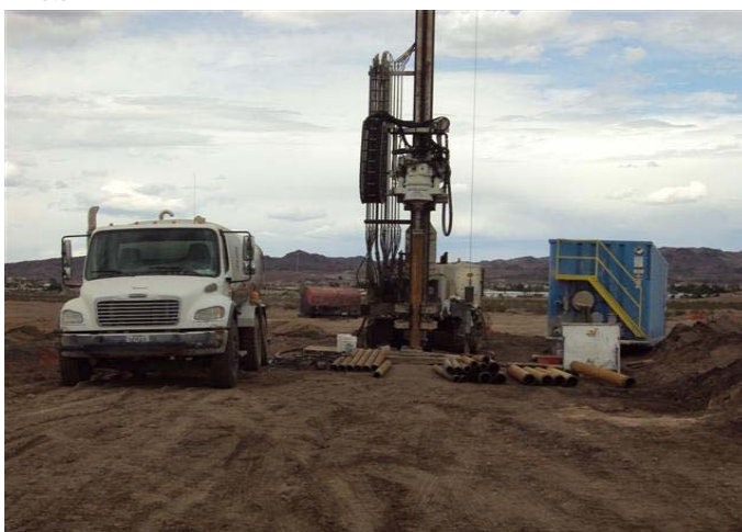
Eastside: GES/Eagle Well installation.
