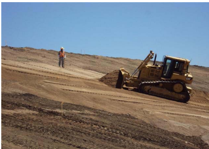
CAMU: Phase IIIA, South slope, interim cover placement.
