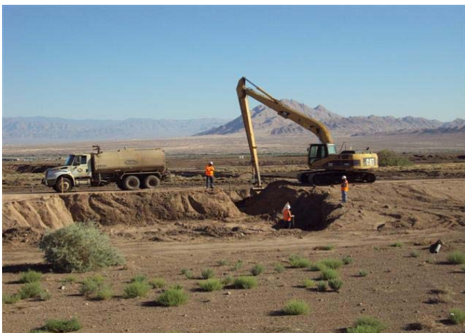
Eastside: Southern rib, exploratory trenching.
