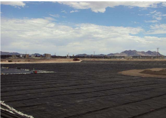
CAMU: Phase IV, liner installation.
