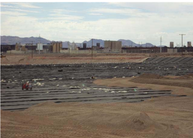
CAMU: Phase IV, liner and operations layer.
