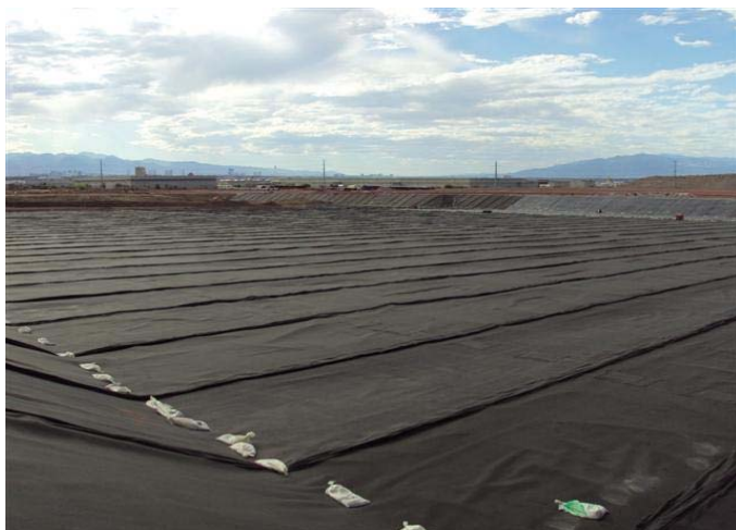
CAMU: Phase IV, Liner installation.
