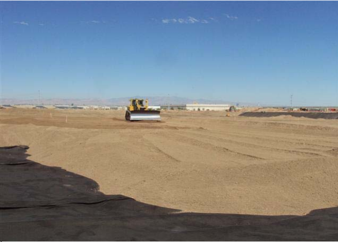
CAMU: Phase IV, Operations layer 1" minus placement.
