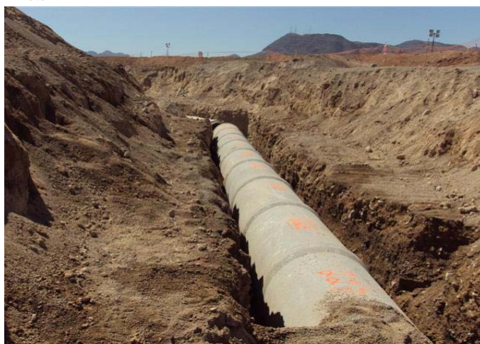
CAMU: RCP, 42" storm drain pipe.
