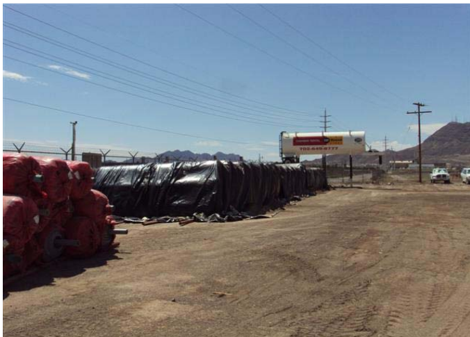
CAMU: Phase V. Geosynthetics staged for installation.
