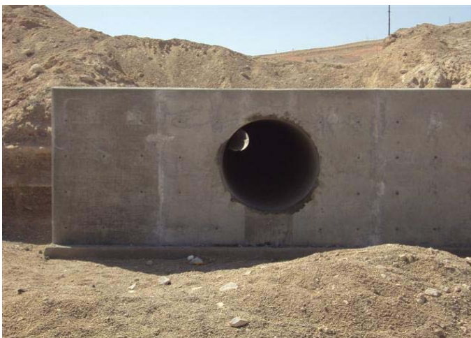
CAMU: Storm drain headwall, into NW Basin.
