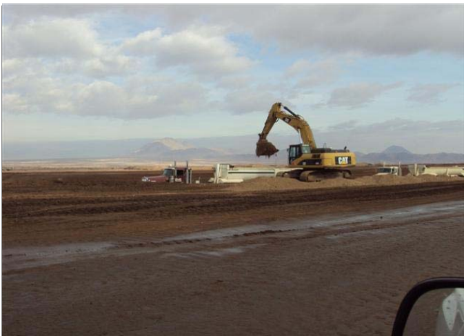
Eastside: HP berm, loading OTR trucks.
