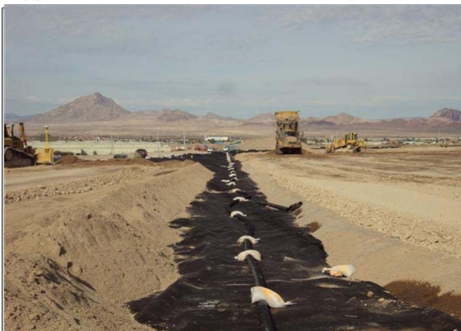
CAMU: Phase I, Phase II, CPE, drain pipe installation.
