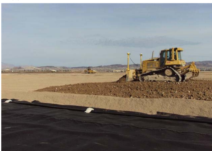
CAMU: Phase I, Phase II, final cover placement.
