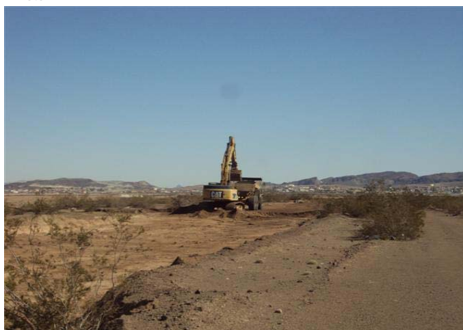
Eastside: Scraping haul road.
