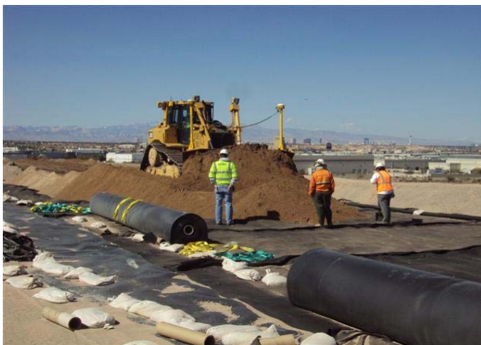
CAMU: Phase IV, monitoring soil placement on liner.
