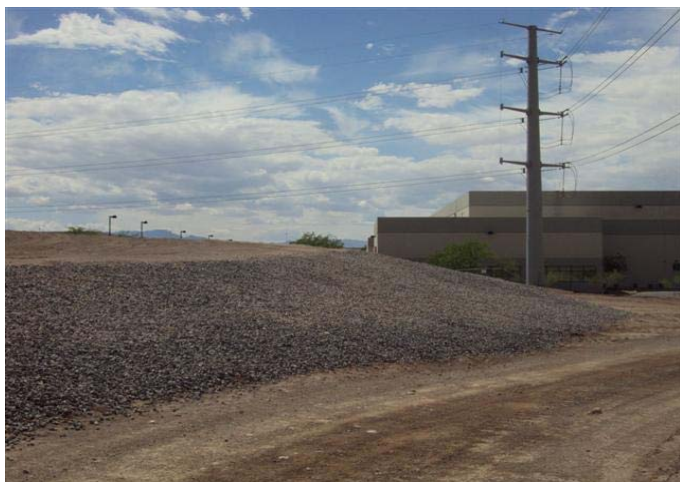
CAMU: BMI North, installing gravel mulch.
