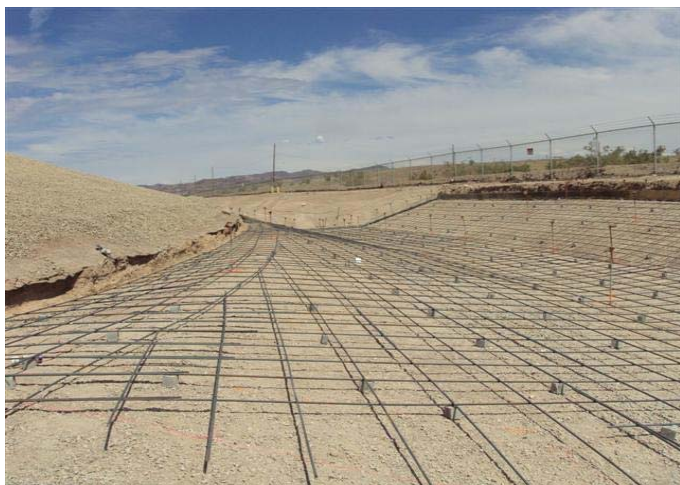
CAMU: Southwest channel concrete preparation.
