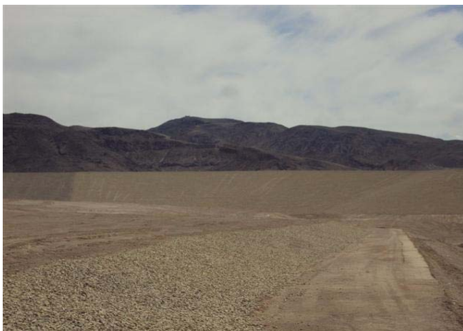
CAMU: BMU North, installing gravel mulch.
