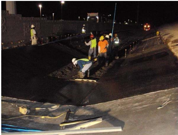
CAMU: West channel, concrete pour and finishing.
