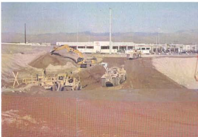
CAMU: Scrapers beginning to remove phase 1 ramp and adjoining soils.
