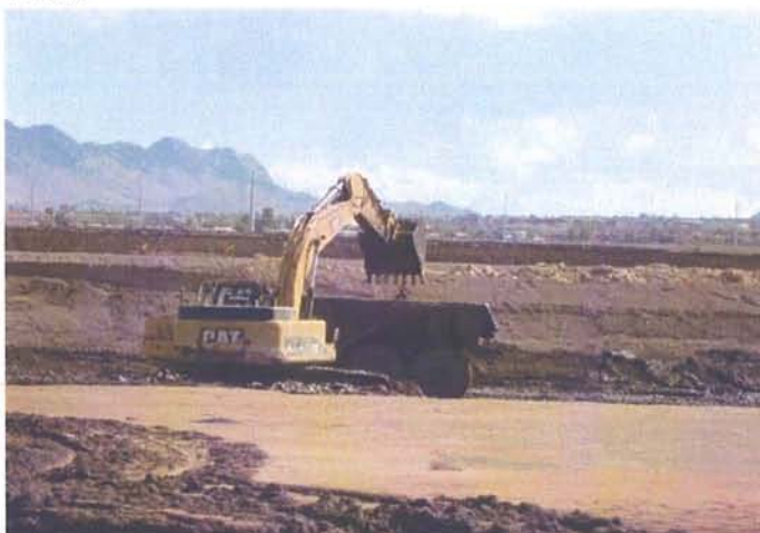
Eastside: Loading out wet soils from SW-10.
