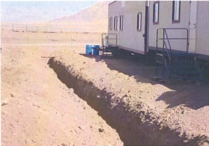
Eastside: Trenching excavated for electrical power..
