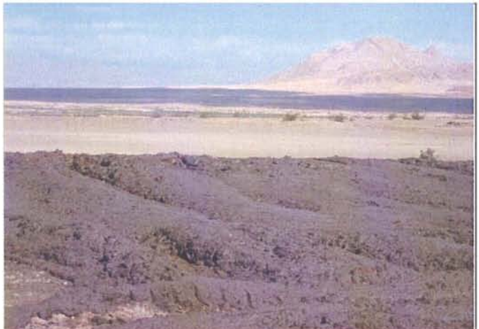
Eastside: Wet soils from SW-11 spread on dry pond. Allowed to partially dry before placing more in order to manage dust.
