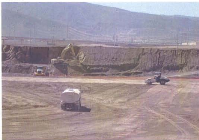
CAMU: Phase 1 western ditch soils being loaded and rolled.
